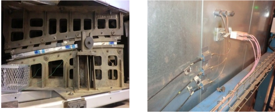
Figure 19. Position of the panel in metallic casing and view of sensors (left) and preamplifiers outside the furnace (right)
