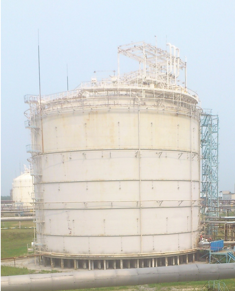
Fig. 1. LPG vessel with ISHM system "Resource-2000"
