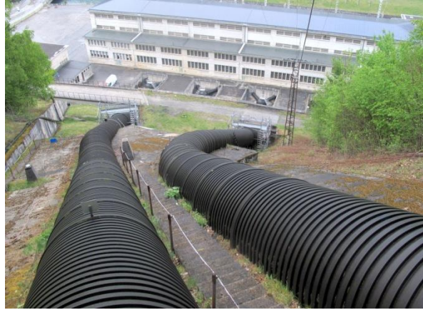
Picture 1: General view of the double hooped penstock
