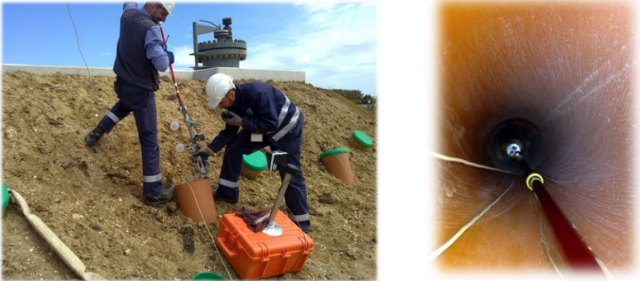
Picture 14 AE Sensors installation through the pipes
