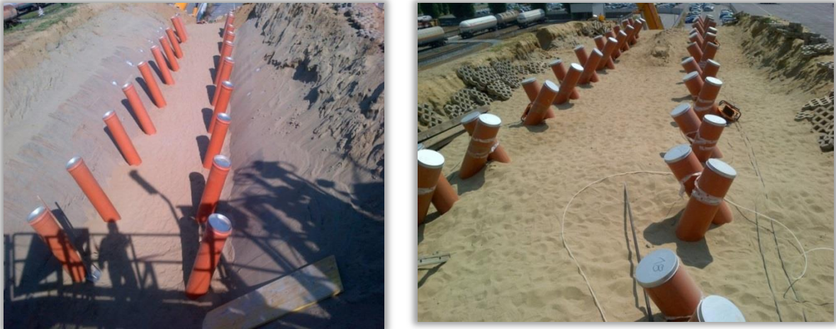
Picture 12 Stepwise pipe installation and sand restore
